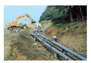
FW SAFETY PIPING DN 100/125, DN 300/350, 3,600 metres, transporting kerosene and diesel oil
